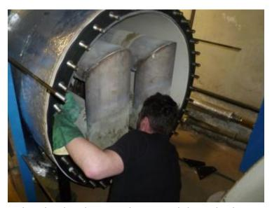
Following the acid wash of the heat exchangers, the gasket was checked for integrity, the hatch rebolted, the cylinder filled, disinfected and returned to service with fresh water.
