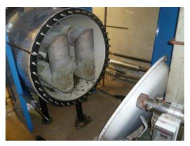
After isolating the cold feed and primary flow to the cylinder, it was drained and the side hatch unbolted as shown.
